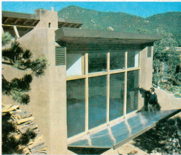
Santa Fe house equipped with reflectors to hold in heat at night Conservation, however limited, is becoming a hopeful factor.
