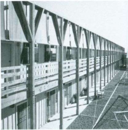
Wood-beam walkways and colored canvas sunscreens "soften" the facades of the metal buildings.
